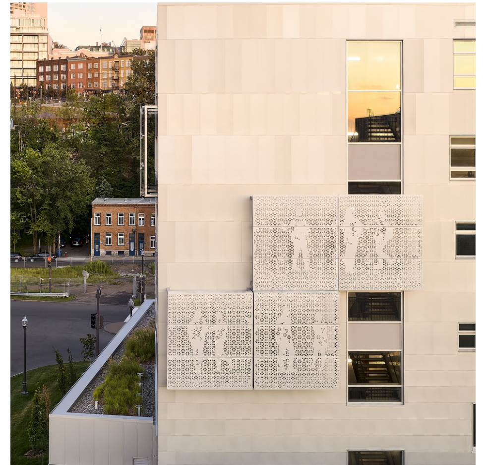
On the facade of the Lauberivière organization's shelter, Lafond-Côté architects developed perforated aluminum panels in collaboration with an artist. They filter the light and provide a level of privacy in particular spaces. (see practice 4.2 a), p. 56)
