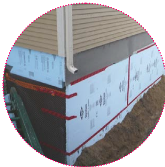
Example of exterior insulation of foundation walls.
