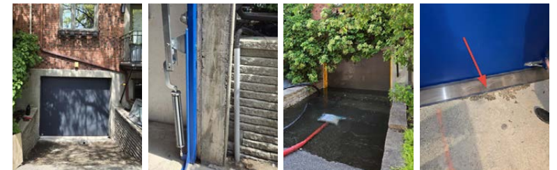
Tests conducted by the City of Montreal in partnership with Écohabitation.
