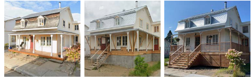
Before elevation work
