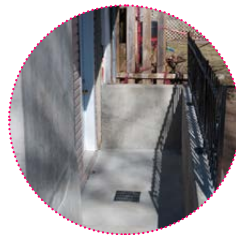
Post-intervention low wall and access stairs installation
